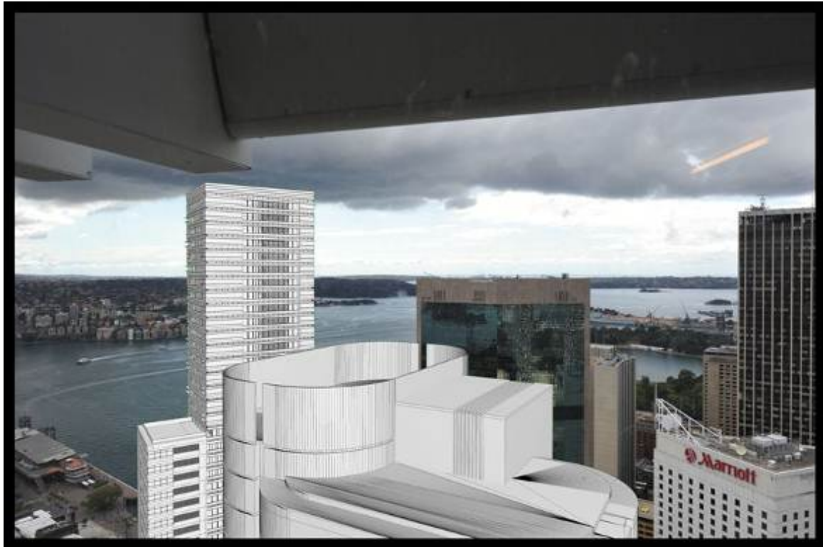
Figure 34 – Outlook from further south along the north east facing curve of Level 43, Grosvenor Place – approved building at 1 Alfred Street and proposed building
