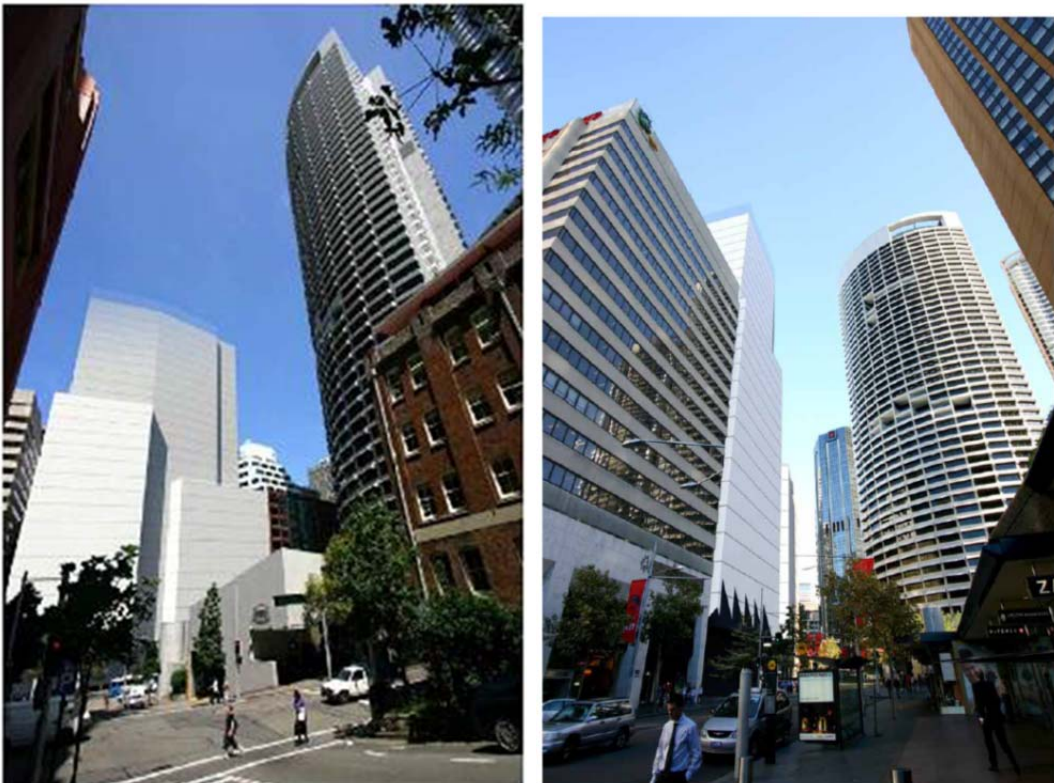
Figures 7 and 8 – views of approved 110m tower envelope looking east along Essex St (left) and looking south along George St (right)
