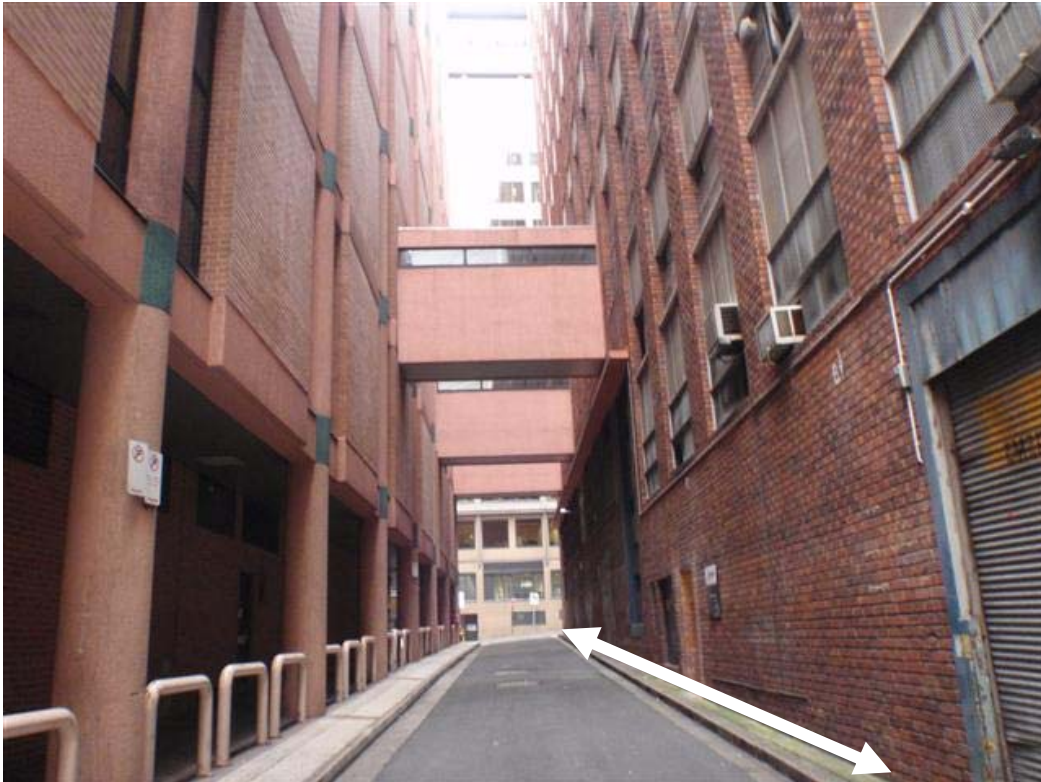
Figure 5 – The building at 4 Dalley Street on the right. The lower parts of the building are occupied by the telephone exchange on a long term lease.
