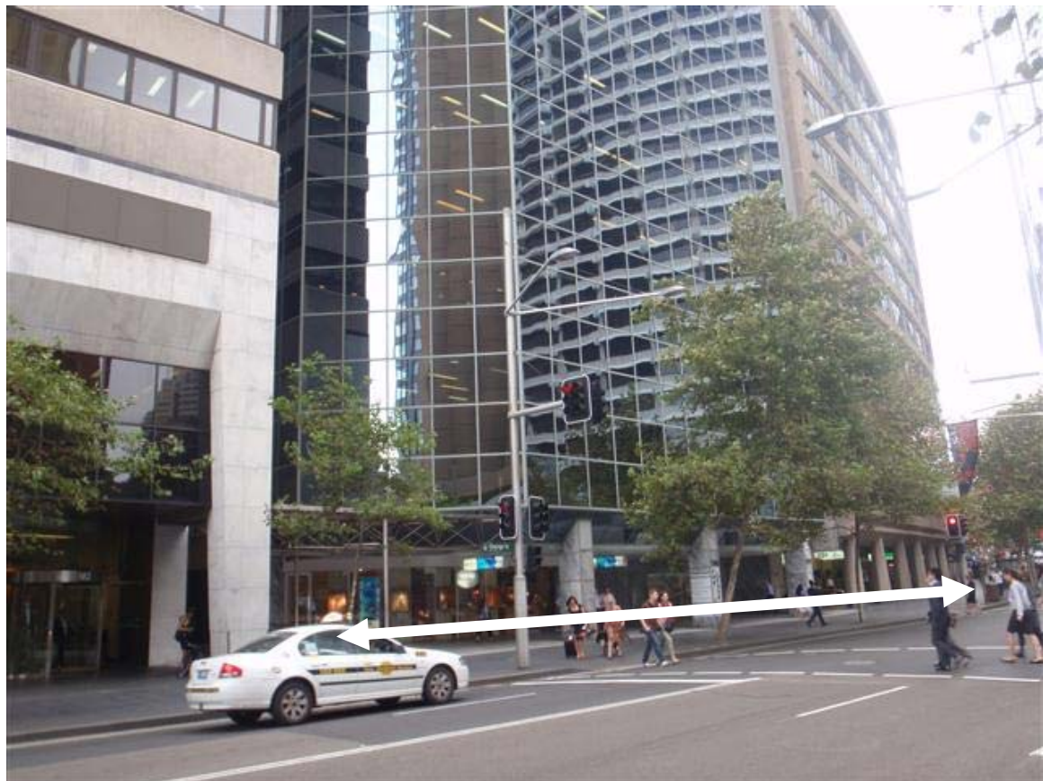
Figure 4 – The buildings at 188-194A and 196-208 George Street
